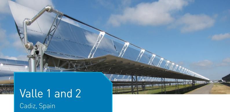
Valle 1 and 2 are adjacent concentrated solar power (CSP) plants located in Cadiz, Spain that feature parabolic trough solar technology combined with thermal storage system.
