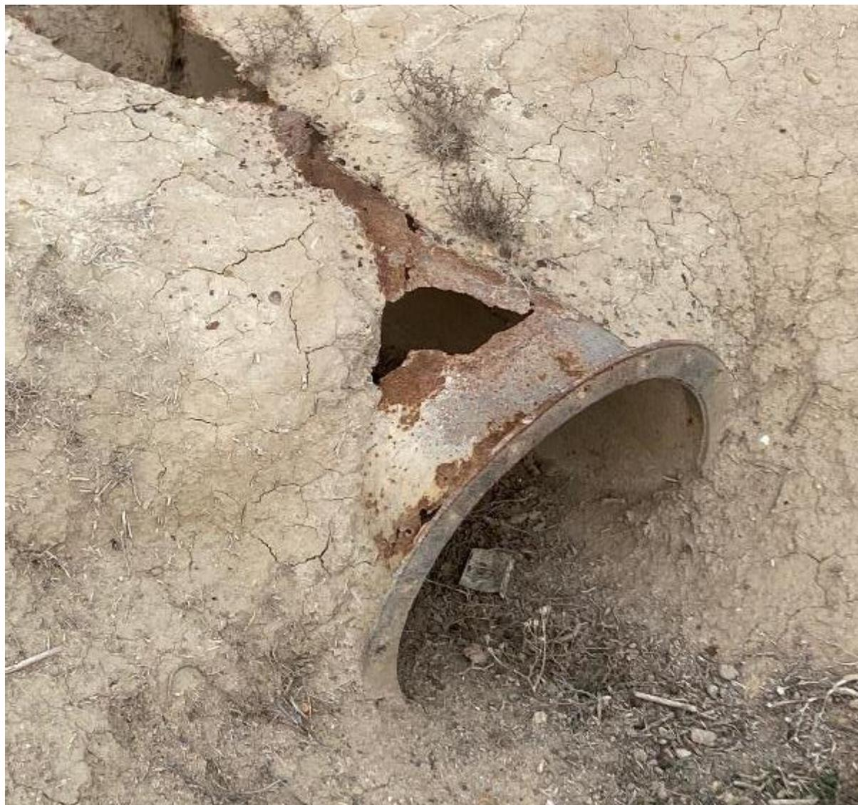
**Figure 3-5: Culvert on irrigation ditch no longer in use**
