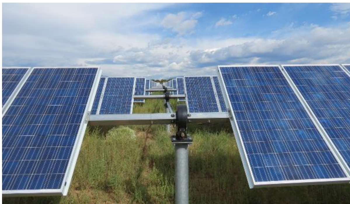
Figure 2-13: Typical PV Facility, using Tracking System
