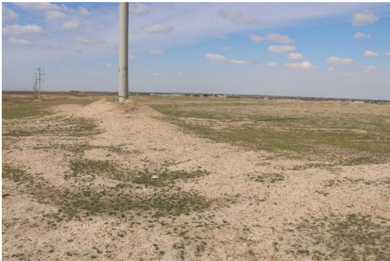
Figure 6-34: OHL Tower built on the remains of the fortress wall
