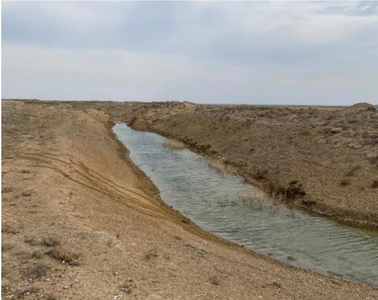
Figure 2-10: Drainage channel (collector) on eastern boundary of site
