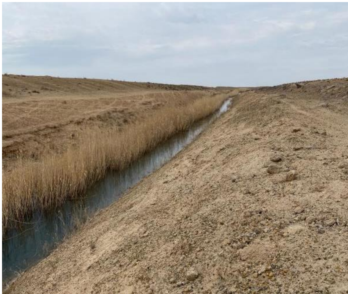
Figure 2-11: Drainage channel (collector) on western boundary of site
