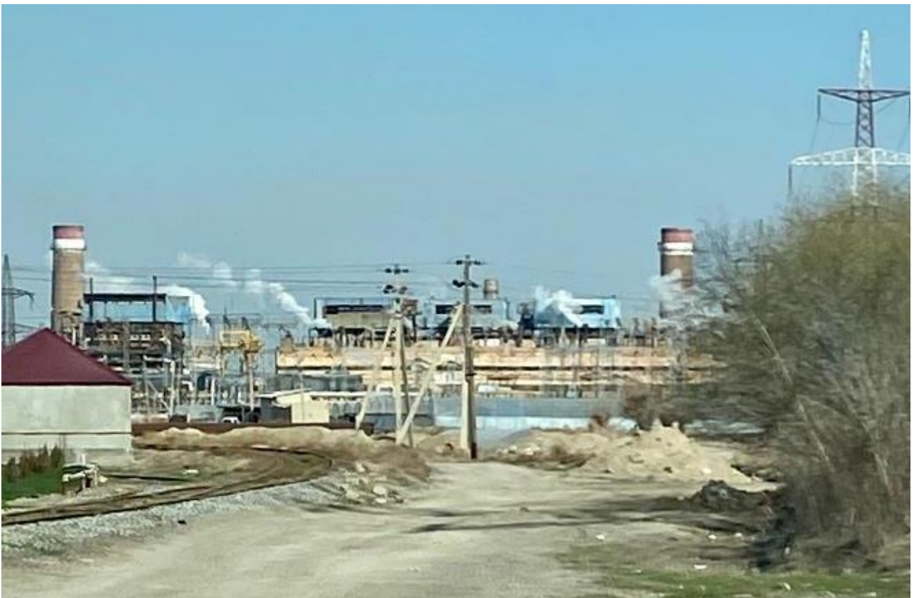
Figure 6-16. LCA 04 Navoi and Environs – View of Coal Fired Power Station from the M37
