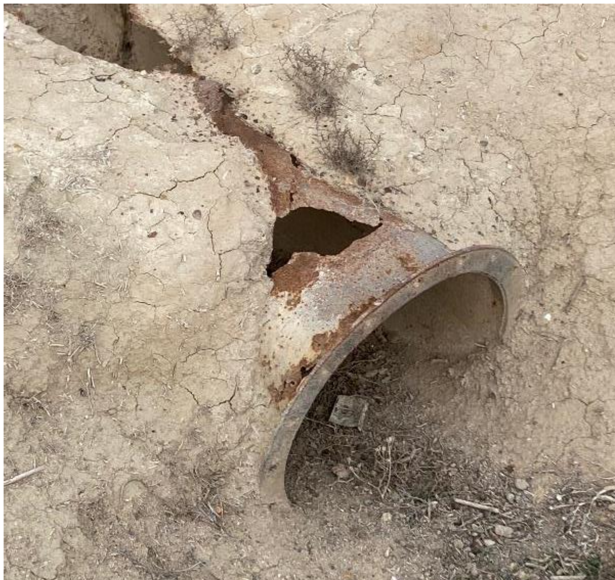
Figure 2-5: Culvert on irrigation ditch no longer in use
