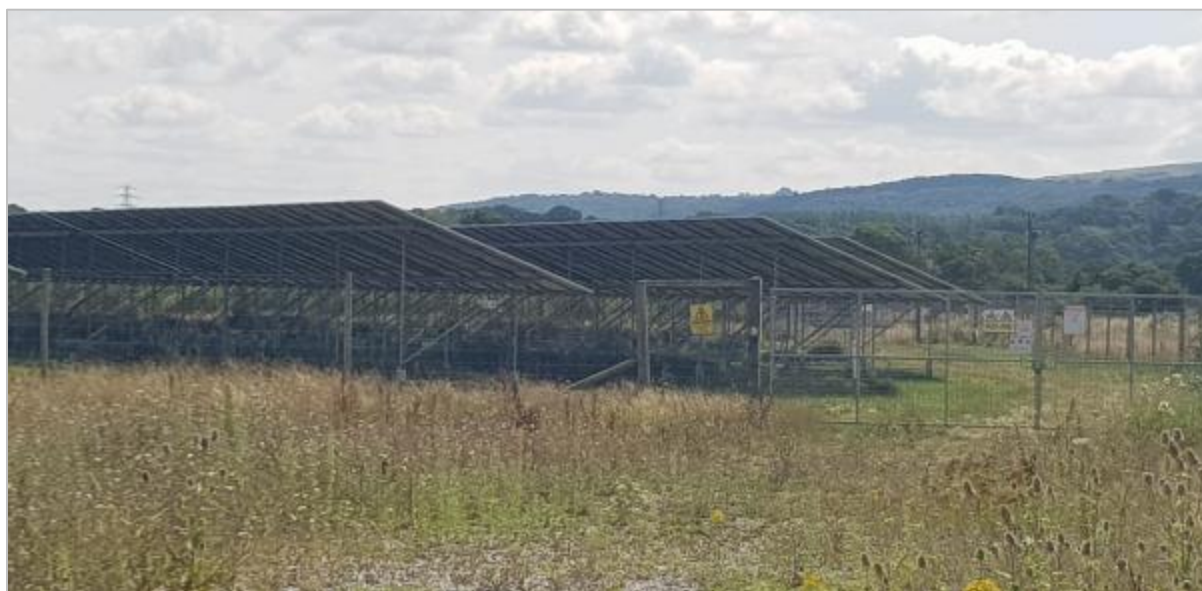
Figure 2-20: Typical Fence and CCTV System at a UK PV Facility
