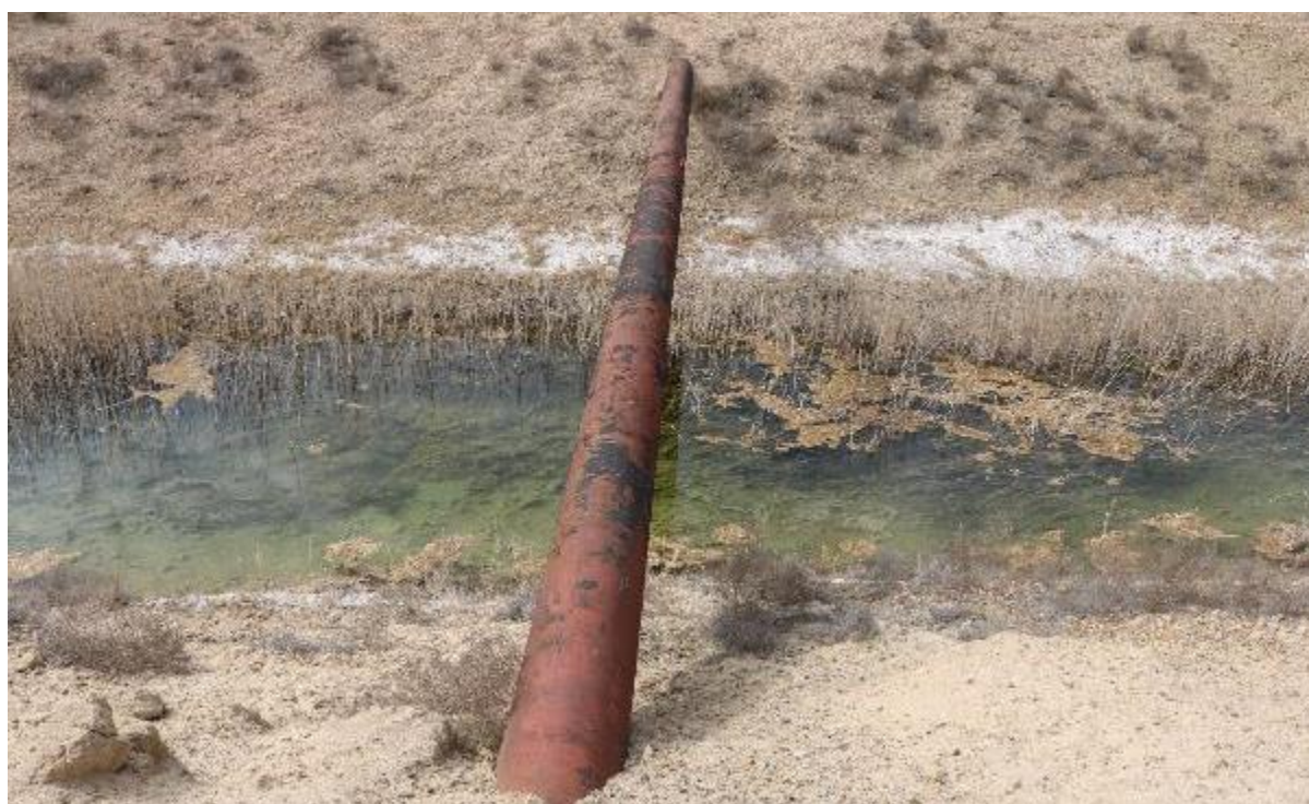
Figure 6-9: Water pipe crossing (March 2020)
