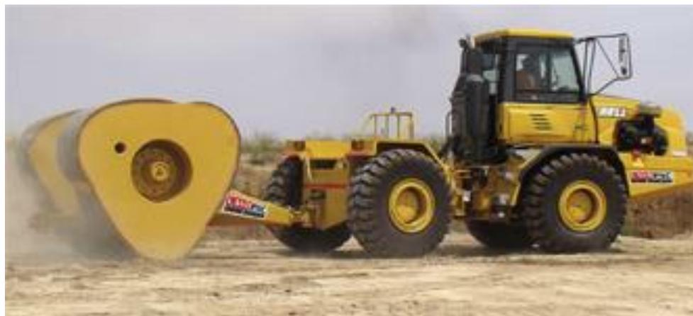
**Figure 2-17. Rolling dynamic compaction (RDC)**
