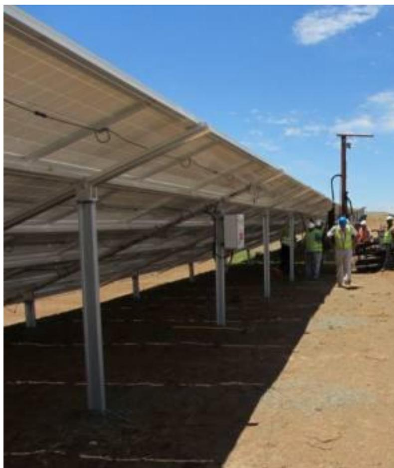
**Figure 2-8. Example of fixed tilt solar panels on H-style steel piles**
