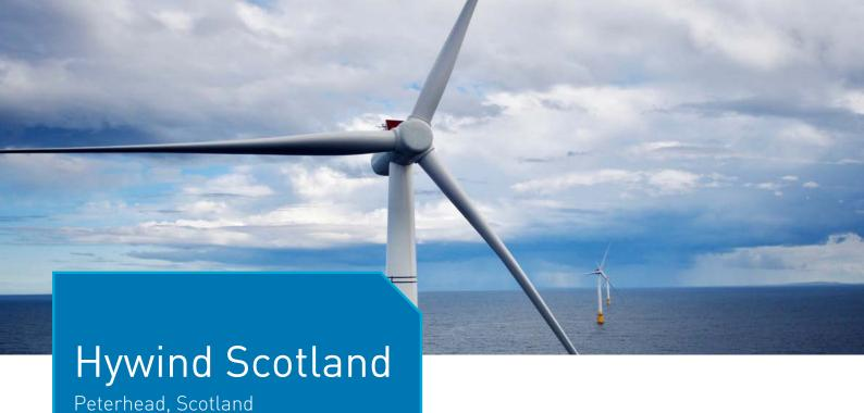
Hywind Scotland is the world's first commercial- scale floating offshore wind farm. Located 25km off the coast of Peterhead, Scotland where the average wind speed is 10 metres per second, the 30 megawatt (MW) farm is a GBP210 million project.
