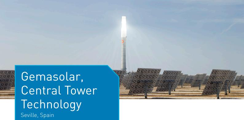
Gemasolar is the world's first utility-scale solar power plant to combine a central tower receiver system and molten salt storage technology enabling electricity supply 24 hours a day. The plant has an installed capacity of 20 megawatts [MW].
