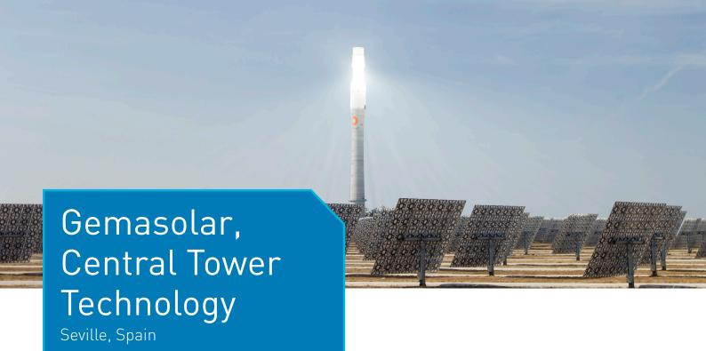
Gemasolar is the world's first utility-scale solar power plant to combine a central tower receiver system and molten salt storage technology enabling electricity supply 24 hours a day.
