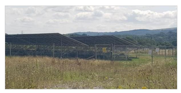
Figure 3-19: Typical Fence and CCTV System at a UK PV Facility
