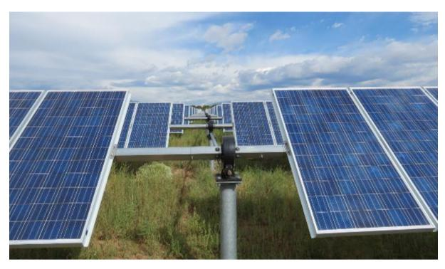
Figure 3-13: Typical PV Facility, using Tracking System
