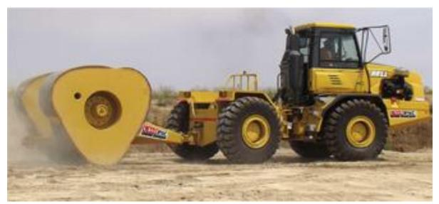
Figure 2-22. Rolling dynamic compaction (RDC)
