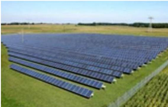
*Figure 6: PV tracking system and inverters (Single-axis trackers follow the sun east-to-west on a single point)*
