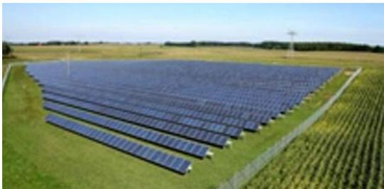
*Figure 7: PV tracking system and inverters (Single-axis trackers follow the sun east-to-west on a single point. NEXTracker)*
