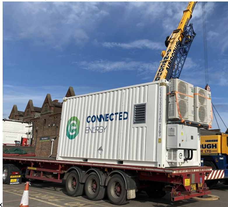
Figure 94: Example of delivery of BESS containers
