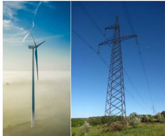
Figure 2. Generic wind turbine and OHTL tower
