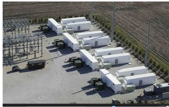
Figure 8: Typical container BESS (external) 1
