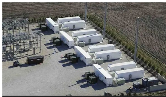
Figure 8: Typical container BESS (external) 2 :
