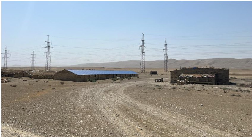
Structure 3 km from nearest WTG
