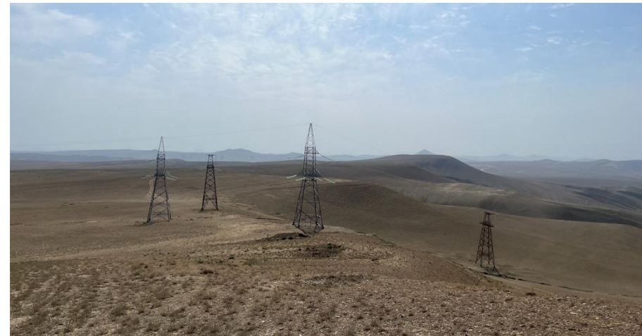
WTG 01-11, view of the existing OHTL
