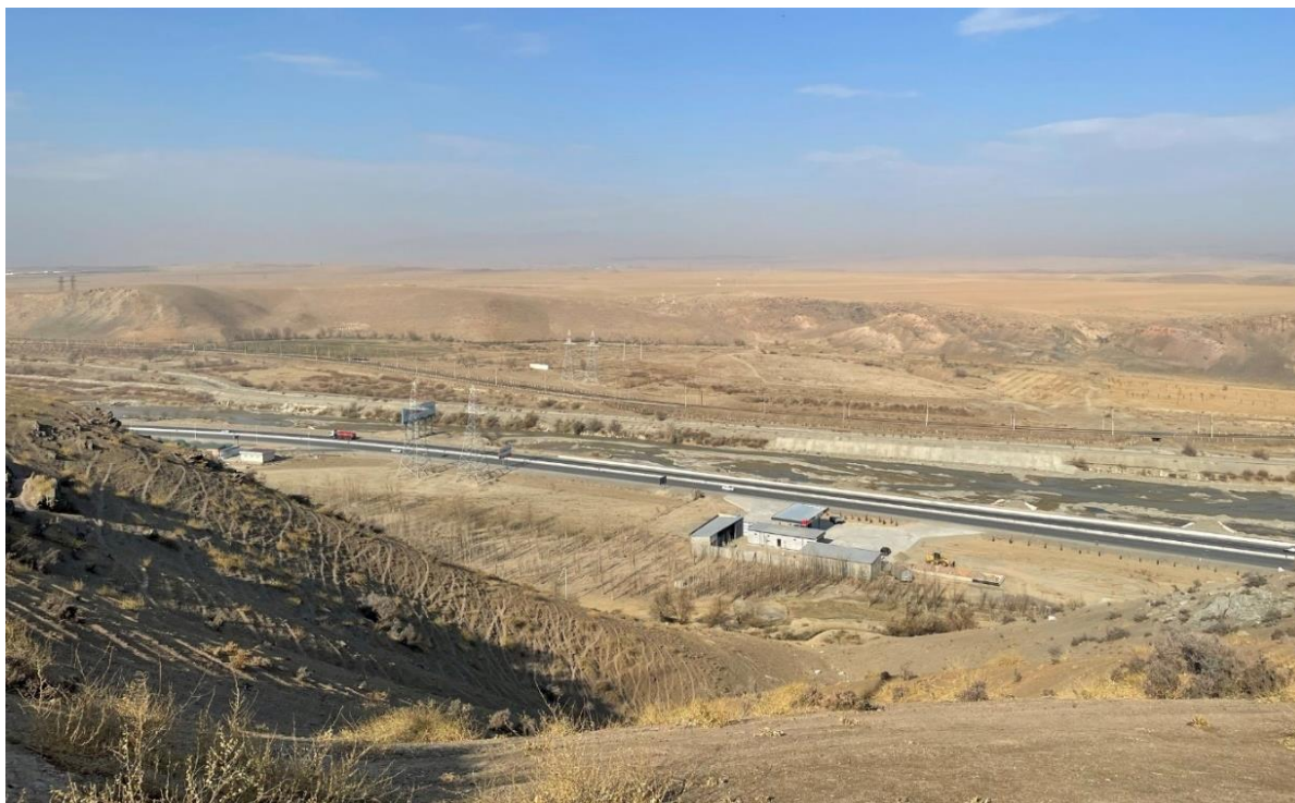
Figure 6-9. Sangzor River valley looking north towards the site
