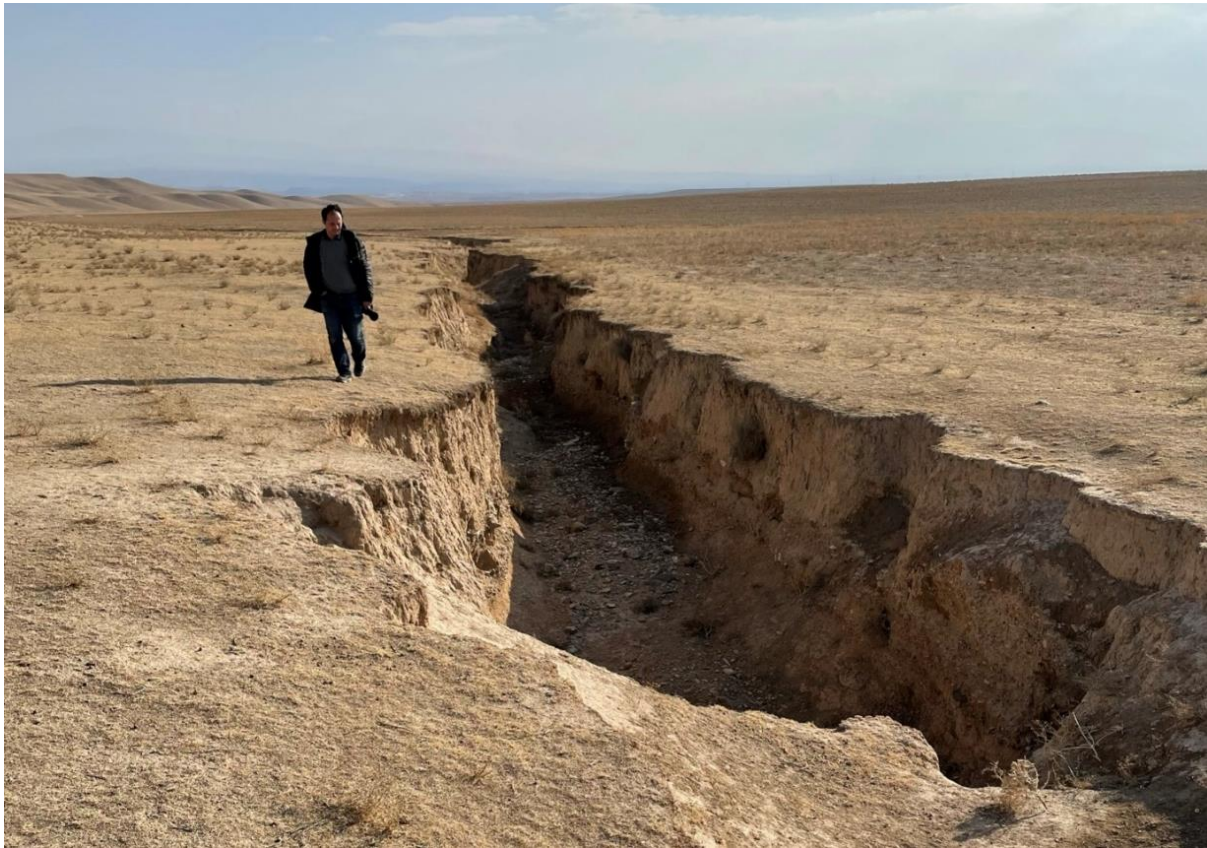
Figure 6-7. Example of gullies found on Site looking south
