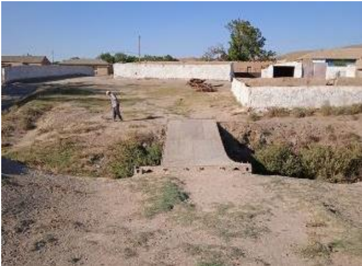
Figure 6-49. Small bridge to primary School 54 in Chayonli village
