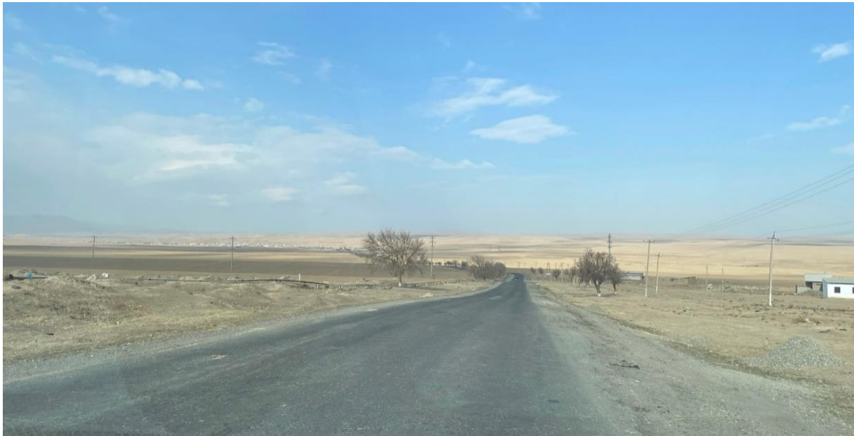
Figure 6-54. Minor road to site entrance at Karakchi
