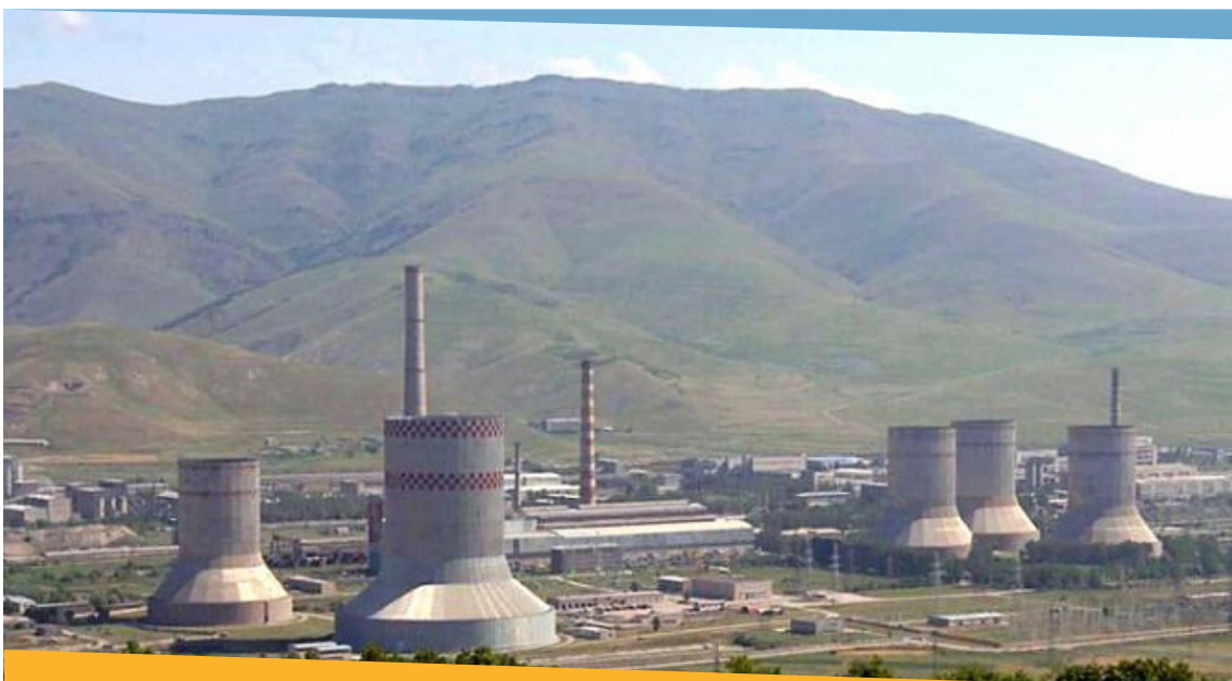
Hrazdan Power Plant
