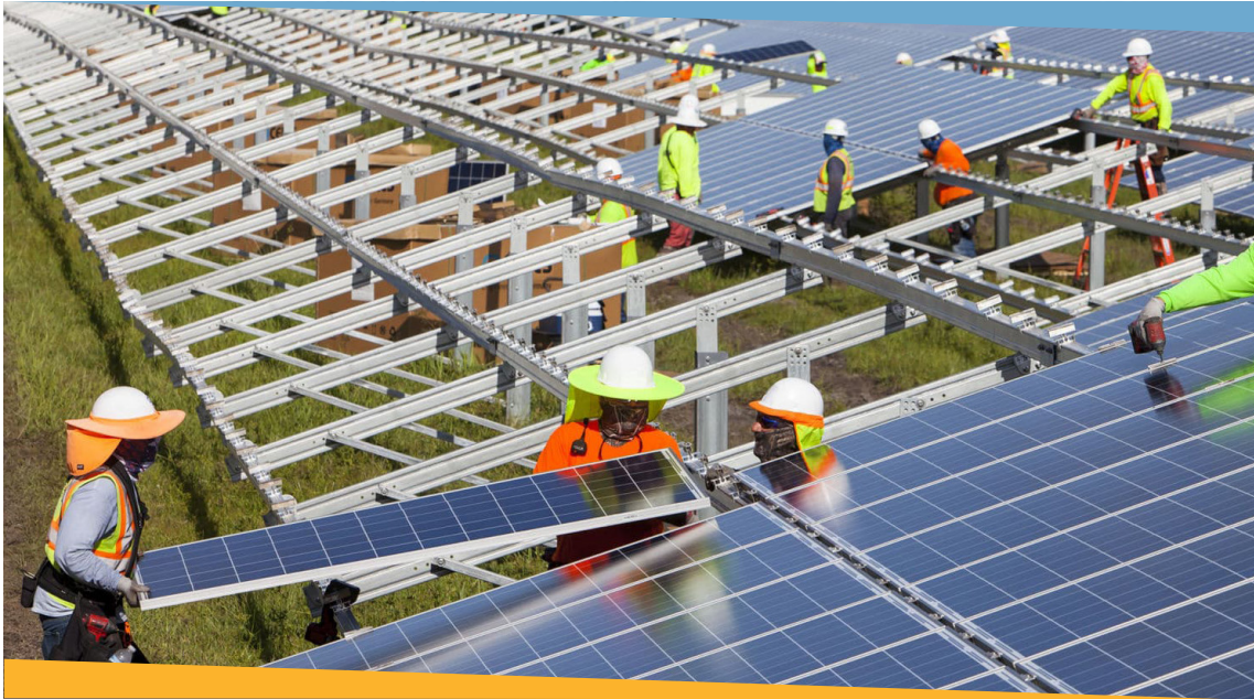
PV Panel Installation
